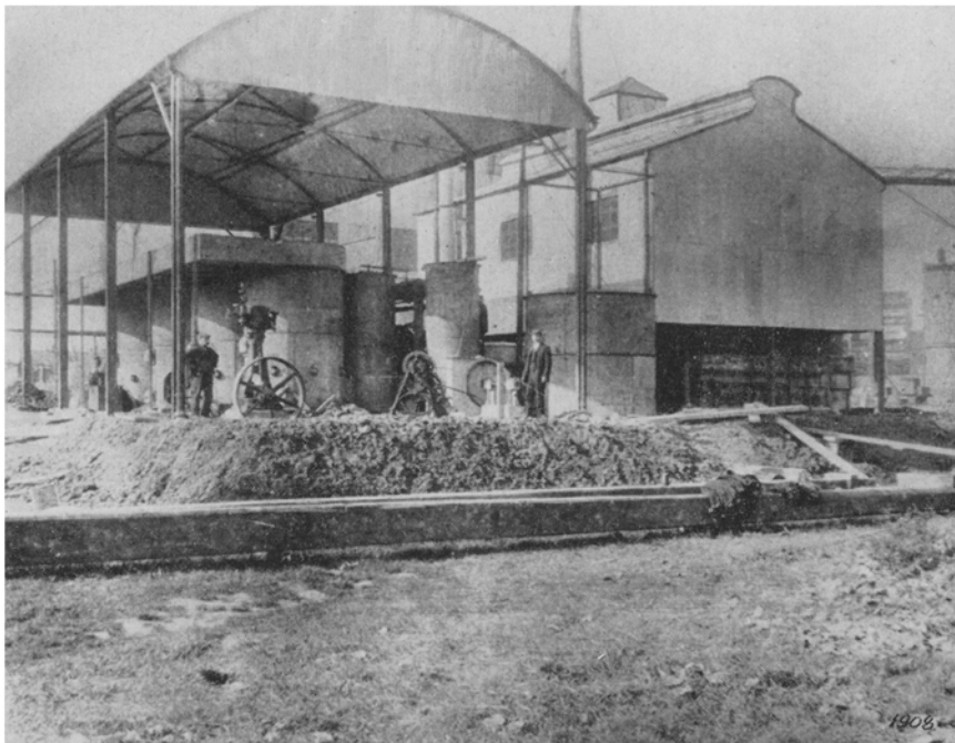
Lane Plant under Construction
